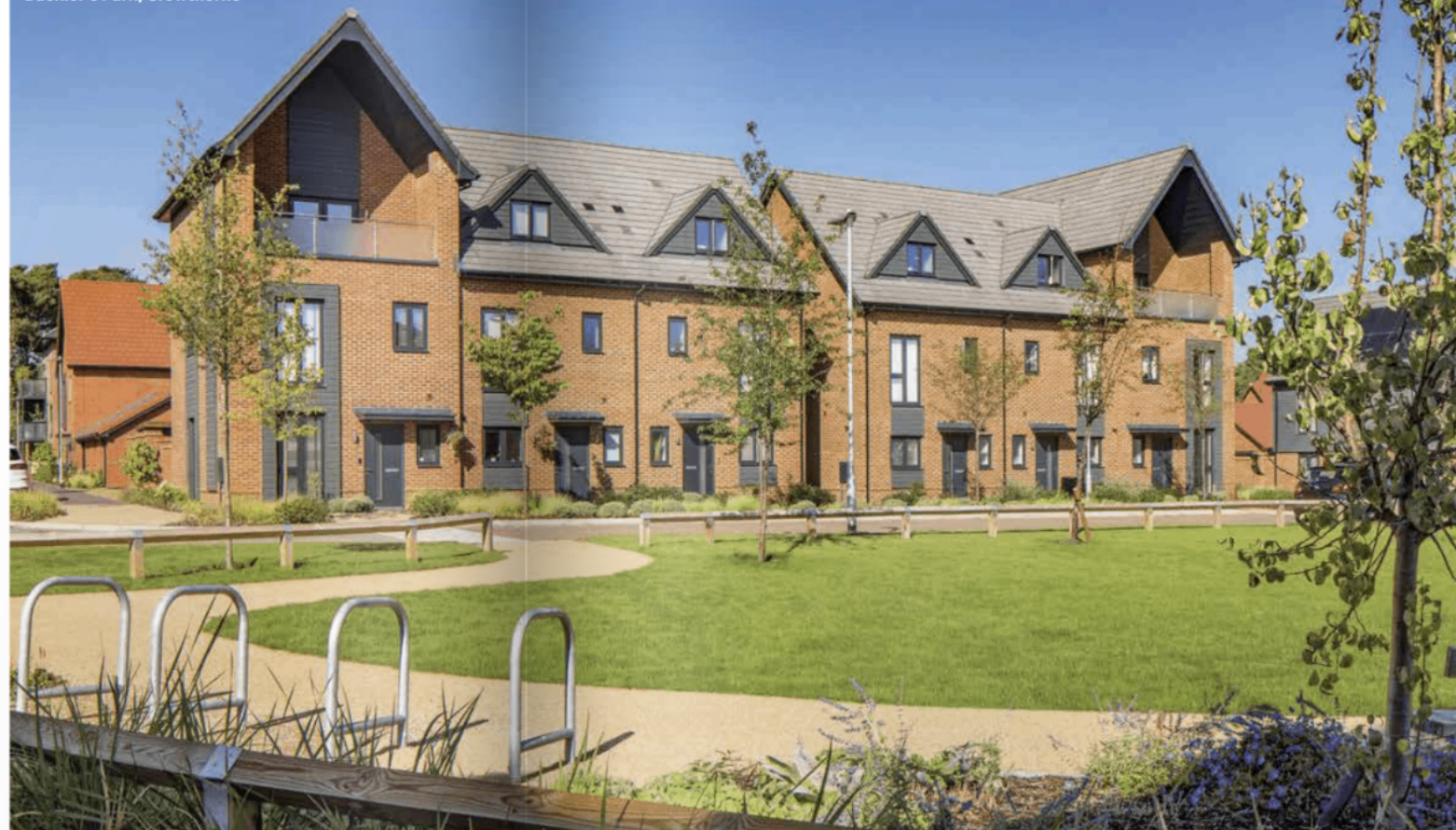
LRG manages the BTR homes at Buckler's Park, Crowthorne
